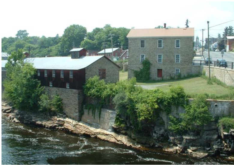
The complex includes the Stone Mill (left) and the Stone Office Building (right), built circa 1850 of local sandstone. The Stone Mill is among the last surviving water-powered industrial buildings in the region. Both are on the National Register of Historic Places.
