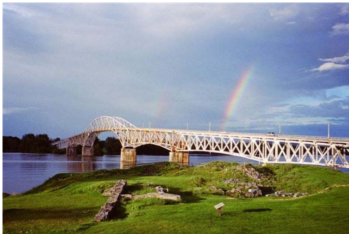
Lake Champlain Bridge. Photo by Tom Hughes
