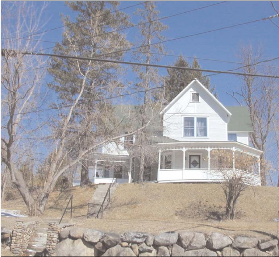
The former home of Hettie Bartlett, at the foot of Mill Hill, overlooking the Jay Covered Bridge site. Bartlett took over operation of the Brick Store across the road, which had survived both the 1856 flood and the withdrawal of the J.&J. Rogers Company from Jay. Besides being a storekeeper, she was also a local judge from 1919 to 1931.
