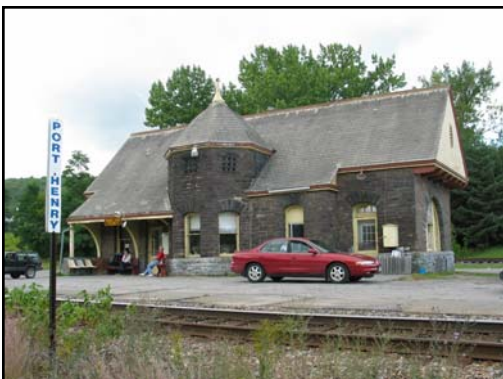
Port Henry Railroad Depot
