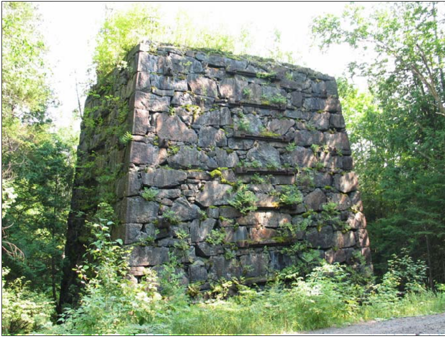
The 1854 blast furnace at Adirondac, the crown jewel of Archibald MacIntyre's ironworks, lay at the end of a toll road built in the mid-19th century from Averyville. Used for less than 4 years, today it rises from the surrounding forest, nearly intact.
