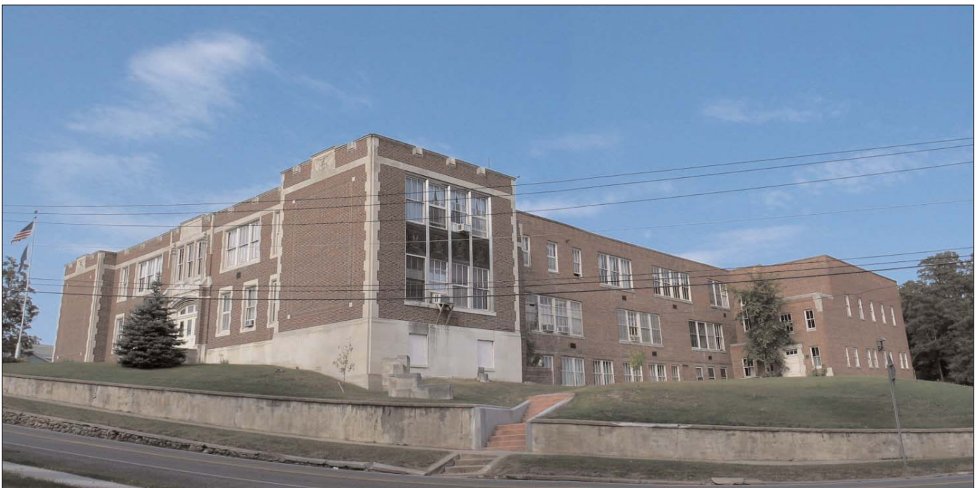
Keeseville Central School, built in 1936, was the third public school built on its Academy Hill site.
