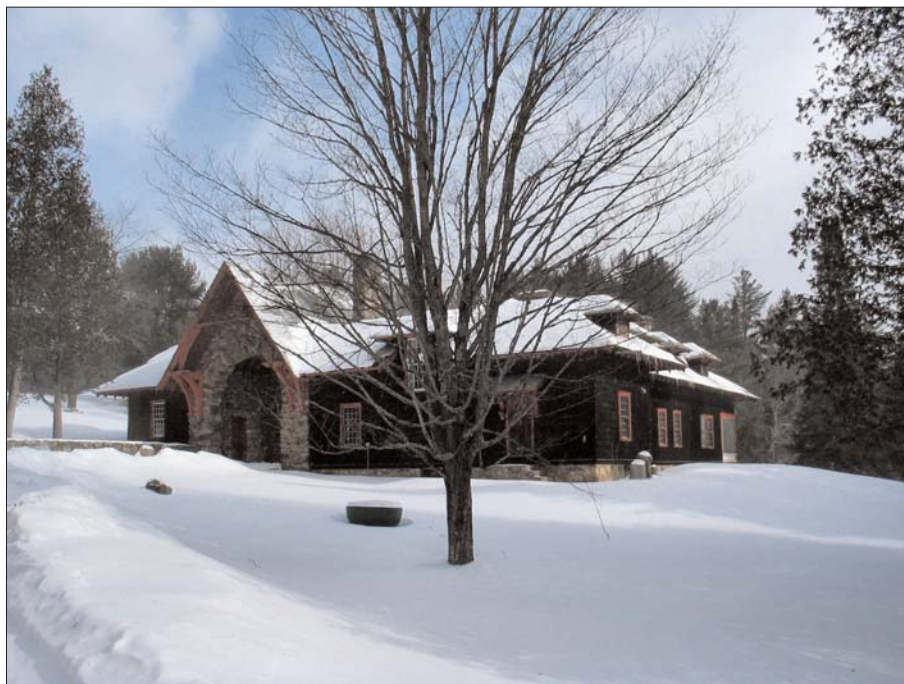
The Gatehouse Lodge at Camp Santanoni
