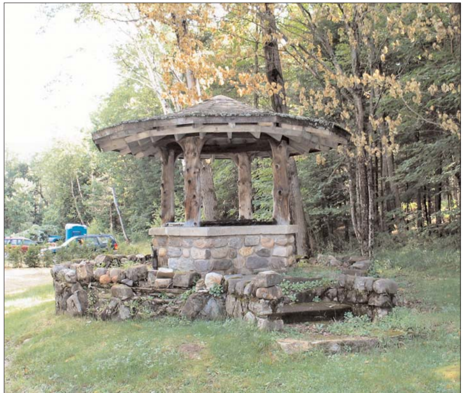
The well at the Caretaker's Complex, White Pine Camp.
