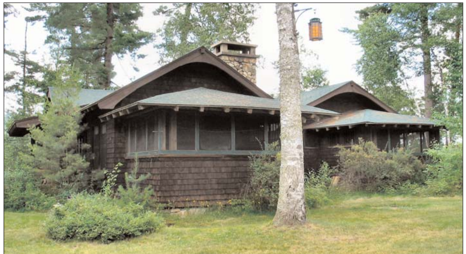
Twin cabins at Northbrook Lodge show a distinctly Japanese architectural influence.
