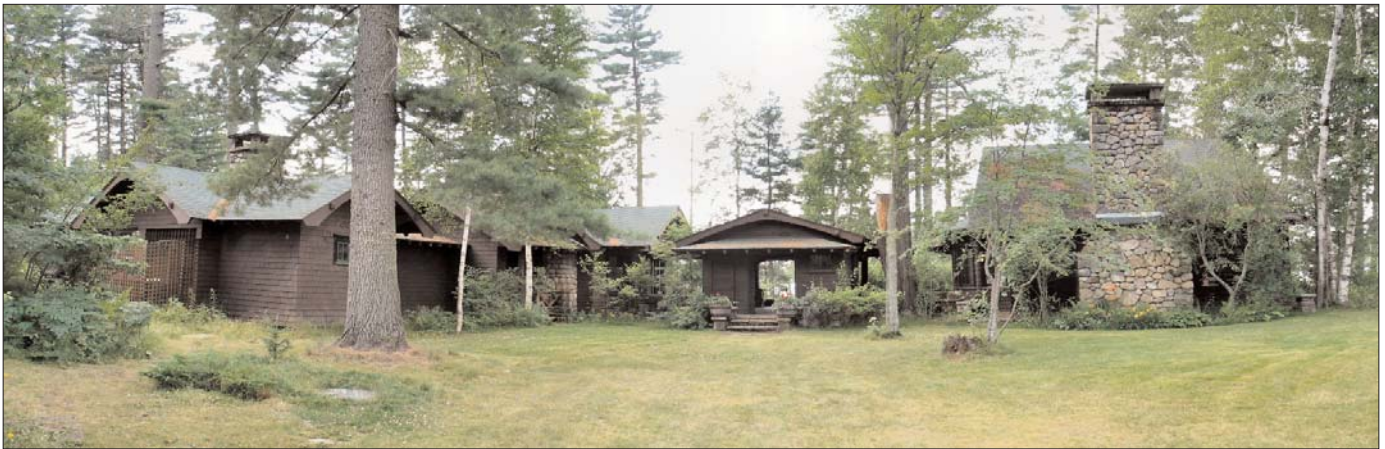
Northbrook Lodge's library and dining room, at either end of this group of buildings, are joined by open, covered walkways, at the center of which stands a distinctly Japonesque entry pavilion.
