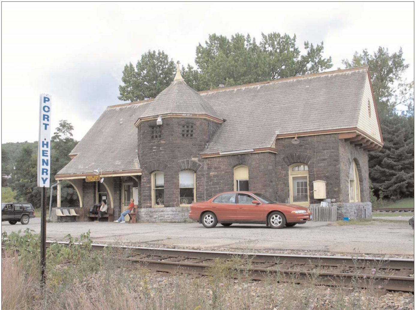
Port Henry's Richardsonian Romanesque train station, built in 1888, now the Moriah Senior Center.
