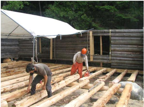
Over the summer, the crew reinstalled stone foundation blocks, built an entirely new floor and sill system, conserved existing logs, and installed new logs, as needed. In addition, several drainage trenches have been put in place in and around the building to allow for proper drainage. To accomplish all this, the existing log walls had to be stabilized and the whole building was raised, in order to replace the deteriorated components of the building underneath.
