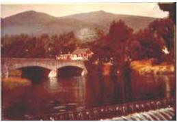
**Wilmington Bridge** (Wilmington, NR/SR). This two-span, stone-faced, concrete arch bridge was built between 1934 and 1935 by C. L. Smith for \$70,375. It was built at about the same time as the Whiteface Veterans Memorial Highway. Both used rough hewn granite as a way of making the structures fit well with their natural surroundings. The 160’ bridge was rehabilitated in the 1990s and is in good condition.
