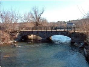
**Frasier Bridge** (Ticonderoga, NR). This two span, stone arch bridge was built over the Lachute River in 1875.
