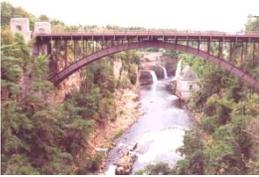
**Ausable Chasm Bridge** (Ausable Chasm, NR/SR). This bridge was built between 1932 and 1934 by Burr Stark of Hadley, New York for \$63,323. It includes a 212’ steel arch span, two 52’ stone-faced, concrete arch approach spans, and other retaining walls and landscape features faced with local sandstone and granite. The bridge was extensively rehabilitated in the 1990s and is in good condition.
