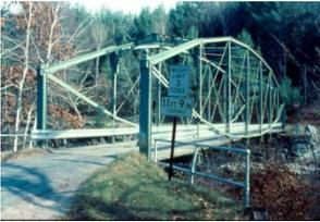
**Walton Bridge** (Keene, NR/SR). This bridge was originally built circa 1890 by the Berlin Iron Bridge Company in Black Brook (Clinton County) and was moved to its present location in Keene around 1925. It is a 96’ long, pin-connected, lenticular or parabolic truss bridge and is one of only about 40 of this type that still survives in the United States. It is presently closed to vehicular traffic but is still used by pedestrians.
